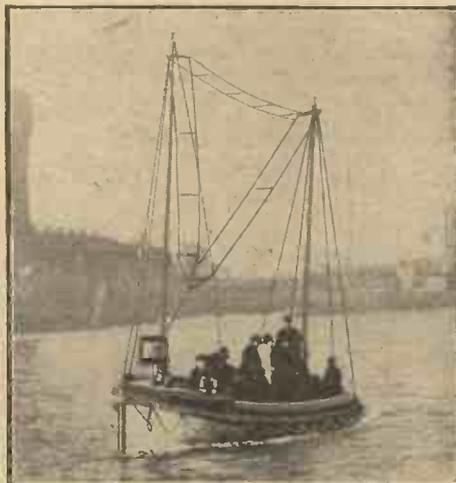
Marconi Installation on a Ship's Lifeboat.
