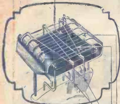
5 resilient filament supports keeping filament in permanent alignment.
