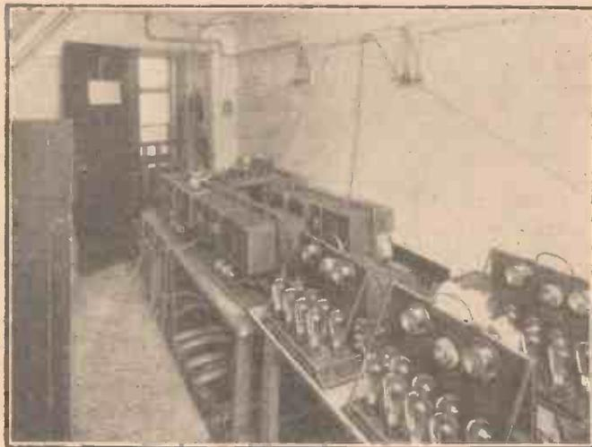
Amplifier control room with Marconiphone power and control amplifiers.
