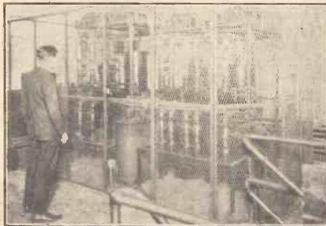
The Kenotron Rectifier Assembly.
