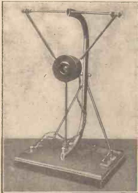
Photograph showing Method of Suspending Microphone.
