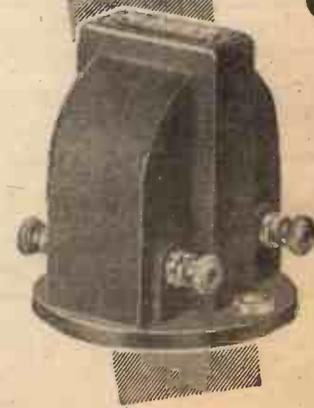
The new British General Midget Transformer created remarkable interest. In accordance with modern practice of economising in weight and space this transformer has been produced in a remarkably small size. The core is of the latest Nickel Alloy (specially treated) and the performance is as good as many transformers at three times the price.
