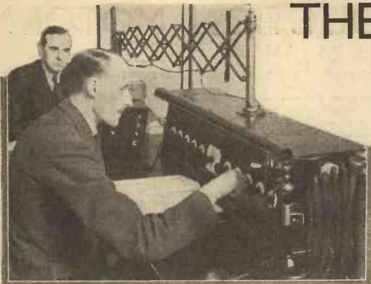
The picture shows the Dramatic Control Panel by means of which the productions of several studios are blended before being actually transmitted
