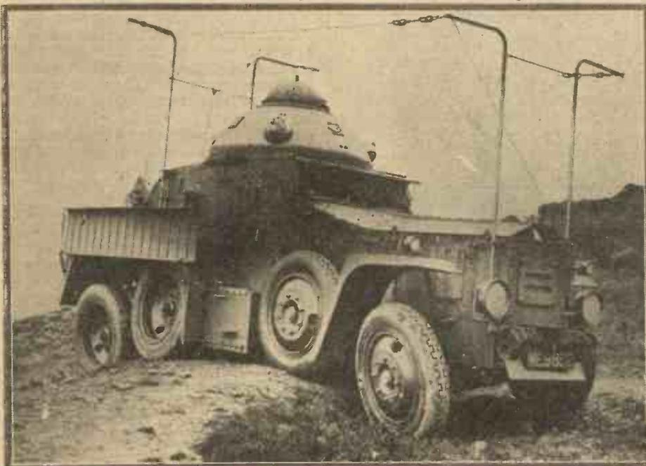
Another radio aid for the Army. Following on the news of the radio-equipped tanks comes this eight-wheeled armoured car, which is fitted up with a transmitter and a receiver, so that it can keep in touch with its objective while on the move. This new monster—a Crossley—is having its eight-wheel chassis and its radio gear tested out in the Derbyshire hills
