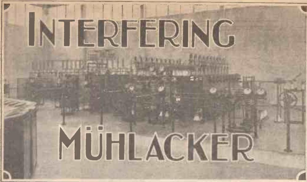
These valves are probably the largest water-cooled valves used for ordinary broadcasting purposes. Whereas at Brookmans Park distilled water is used for cooling (distilled water has a higher ohmic resistance), and is kept in the cooling system, the cooling water being externally cooled by tap water passed over the radiators, at Mühlacker a running water system is used.
