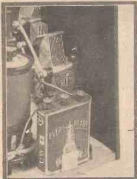
Here is a bias battery inserted in the grid circuit of the high-frequency valve. This improves the H.F. control
