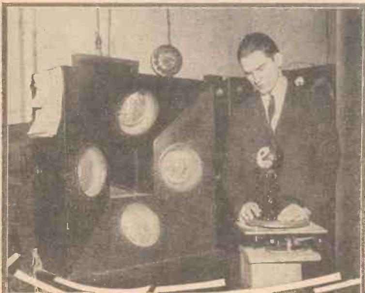
Photo-cells connected to the television transmitter are housed behind this panel with its four windows, and small objects are rotated on turntables before the transmitter so that observers can watch the movement of the image. This is National Broadcasting Co. (American) apparatus
