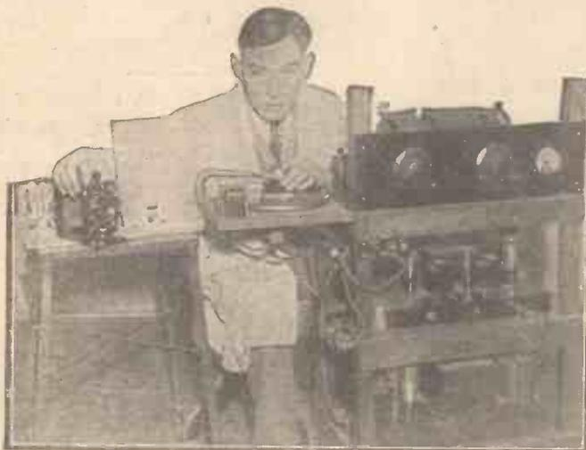
This burglar alarm is switched on by a photo cell-device which can work in the dark. The grammo-radio side of the apparatus is switched on, the receiver of a telephone is lifted off its hook and the record rings up the police! At the same time a powerful light is switched on and the camera at the left takes a "snap" of the eavesdropper
