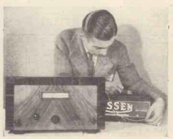
Connecting up one of the high-capacity Lissen high-tension batteries, to the Crusaders' A.V.C.4, a set that gives its best results only with the right type of power supply
