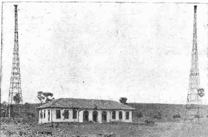
A view of the transmitting station with its T-type aerial
