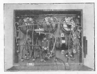
Fig. 64c.—Photograph of Back of Panel showing Wiring.
