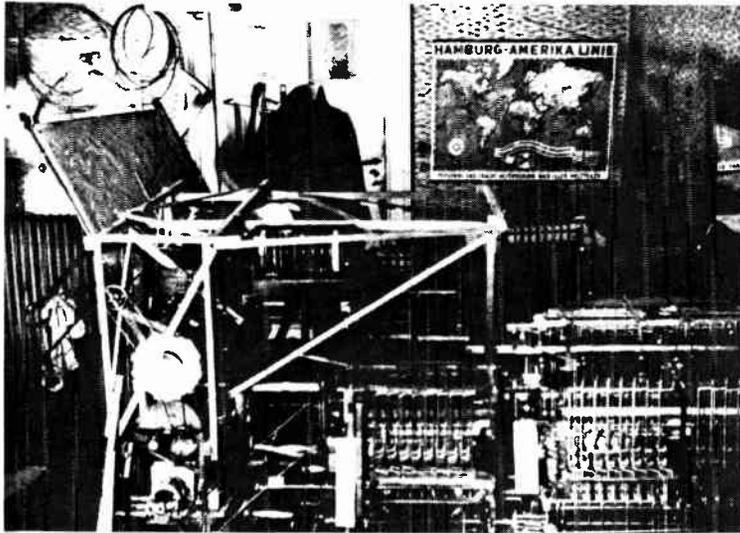
*Fig. 13. This relay-switched digital calculator was built by Zuse in Germany in 1936. (This photograph has been included because of its historical interest – unfortunately the original print is of border-line quality).*
