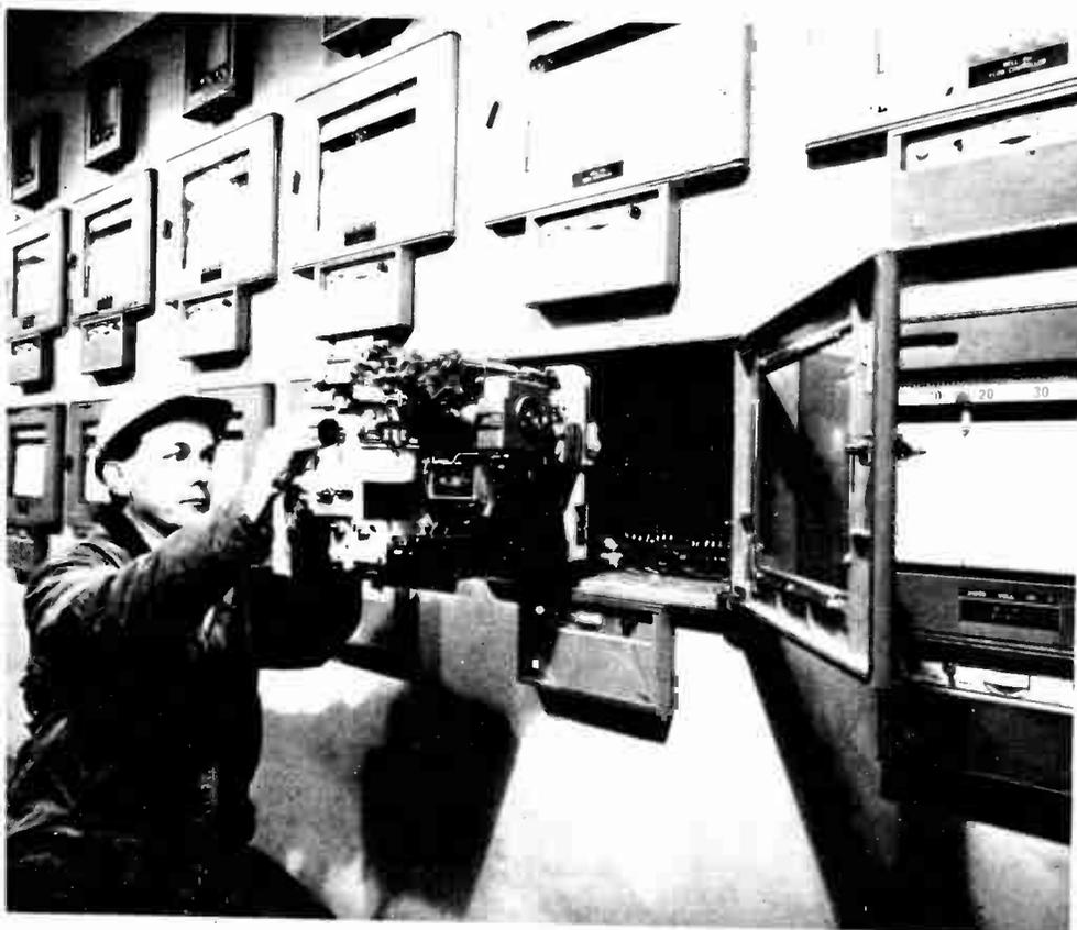
Fig. 1. Chart recorders are used in many varied applications. The panels of this control room contain a number that are used by the operators to see how the process is behaving.
