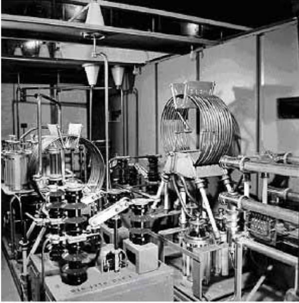
Picture 11: Third Programme transmitter at Daventry: combining circuits, c1950
