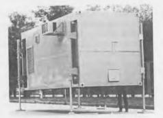
One of the containerised transmitters half fail, the other half carries the entire output.
