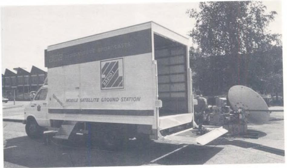
The transportable up-link, as rigged for tests at Concord Road in mid-June. In normal use, the dish aerial and associated equipment will sit on the tailgate of the OB vehicle shown.
