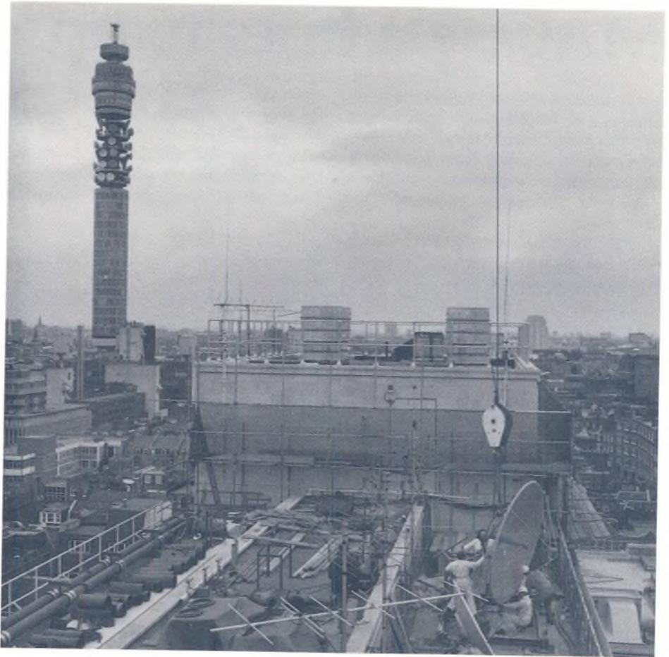
A giant mobile crane lowers the 3 m dish onto the roof of BH.
