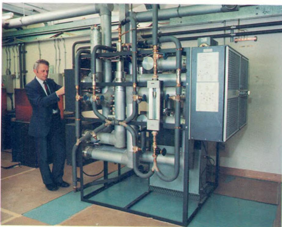
Eric Mitchell operating the high power uhf "feeder switching unit" at Belmont during commissioning. The two large aluminium pipes leaving from the top of the unit are the 50 ohm output feeders, each carrying 15 kW.
