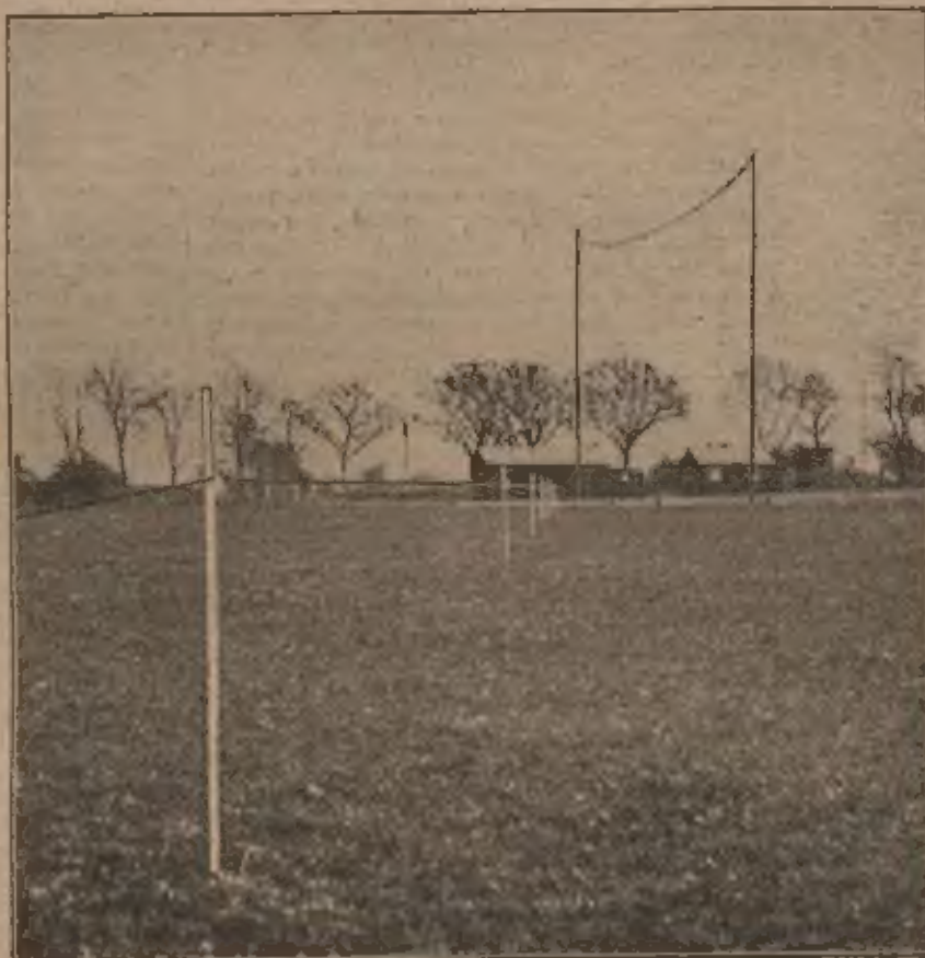
B.B.C.'S RECEIVING STATION AT KESTON.
