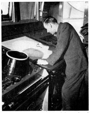
Fig. 9. The plotting screen of the bright display console on the *Canberra*.
