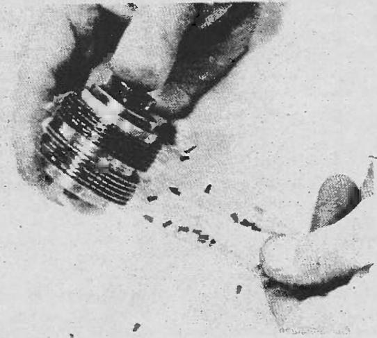
◀ Fig. 2. Cropped-discs assembled on an arbor are used by one manufacturer to control the pattern produced by a knitting machine.
