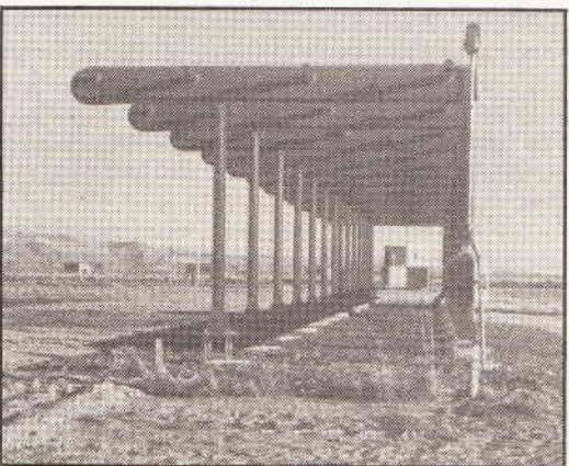
Fig. 7 An ILS localiser aerial, using multiple aeralis to generate the azimuth beam. (Photograph courtesy of Racal).
