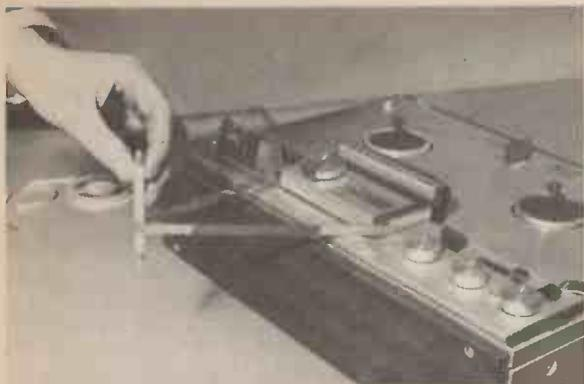
The three photographs on the left illustrate various methods of using a tape loop. The top photograph shows a reversed loop held under tension by passing it around a pencil; this is only suitable for short periods.
