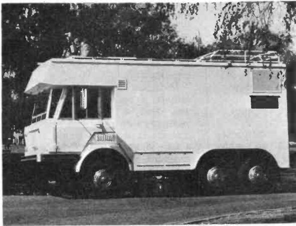
Mini-Mobile OB van introduced by Marconi last year. Note the cameraman with his hand-held portable camera protruding through the vehicle roof.
