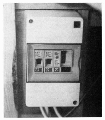
Caravan consumer unit. This has a double-pole switch, an RCD trip and a separate fuse for each circuit.
