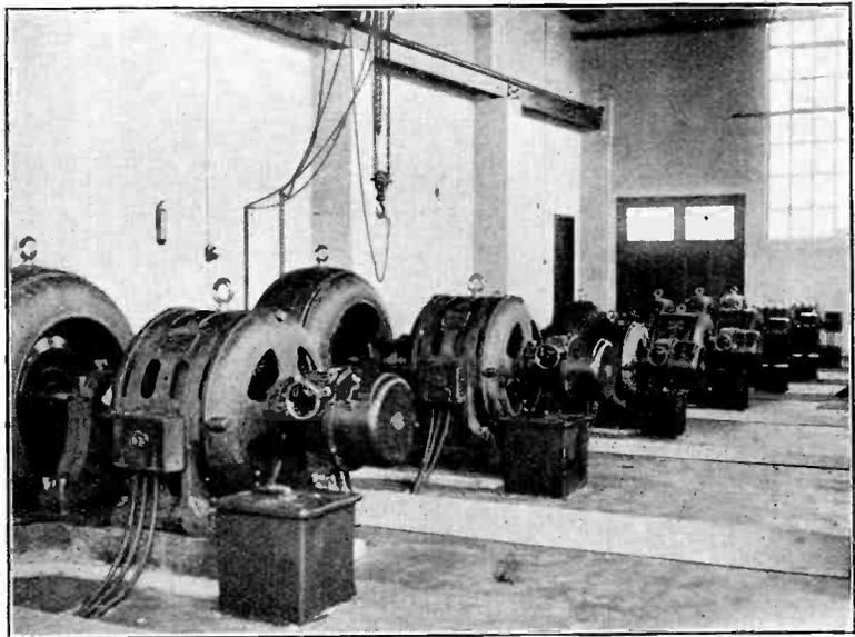
*A view of the Machine Room at Daventry, where are installed three 70 kW motor alternators (two of them are visible in the foreground above); two 25 kW motor alternators; and three 10 kW motor generators.*
