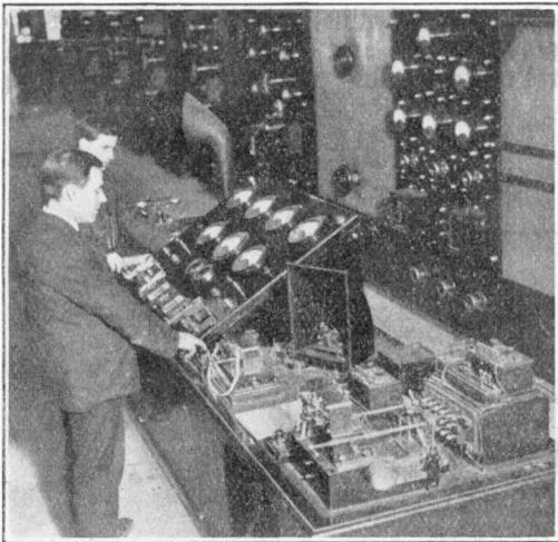
The control table, the central sloping portion containing the switches and meters mentioned in this abstract. To the right of the table is seen the land-line apparatus and to the left is the apparatus for signalling power requirements to the powerhouse. A loud-speaker and wireless recorder also permit checking of the actual signals sent out from the aerial.
