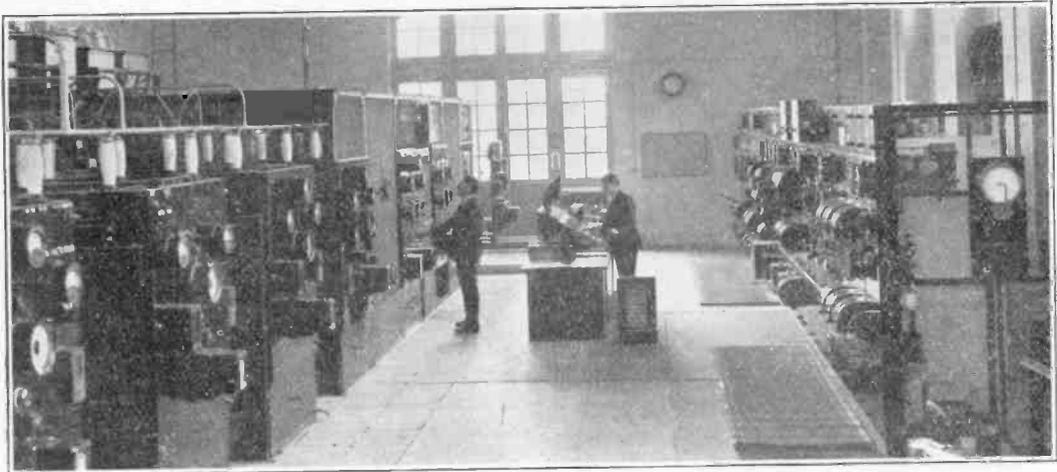
*An internal view of the transmitting room. The control table is seen in the centre of the picture. The second engineer is standing beside the "excitation units," i.e., the 4kW and 50kW stages, as described in this abstract. To the extreme left are some of the power units. On the right is the L.T. switchboard.*
