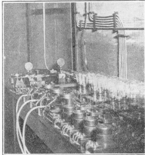
View of a Creed key and pilot keys. These are housed behind the 4kW section of the excitation unit.
