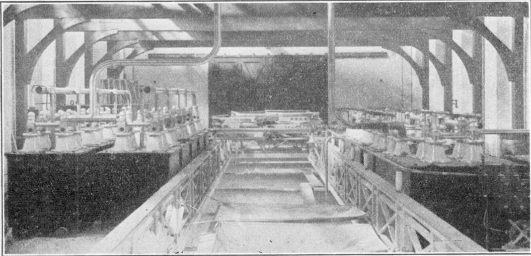
*Mica condensers, oil-immersed, which are being used at the Rugby station. The mica pattern is much less bulky than the condensers of aluminium plates immersed in oil formerly designed by the Post Office for use at Leafield, and the adoption of the mica condenser has helped in the saving of space in the Rugby building.*
