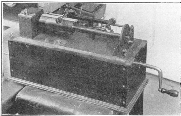
*In the Thorne Baker picture transmitting apparatus a copper plate bearing the image is traversed by a metal needle forming part of an electrical circuit. The receiving and transmitting equipments are exactly similar, and the cylinder on which the picture is recorded by an electrolytic process is kept in synchronisation with the transmitter by means of accurately-timed pendulums.*
