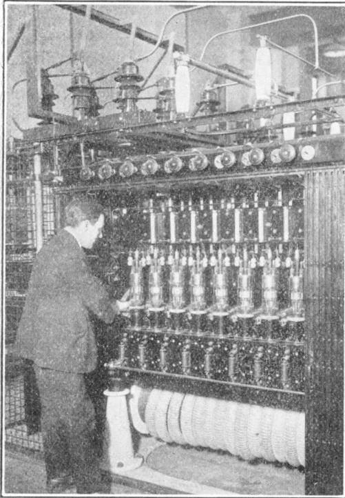
One of the power units with its Bostwick safety gate open on one side. The handles of the filament rheostat for each of the nine valves forming one side of the unit are seen above the gates, while eight of the valves are visible in the photograph, with an overload relay below each. The coil behind the insulator is a rubber water pipe.
