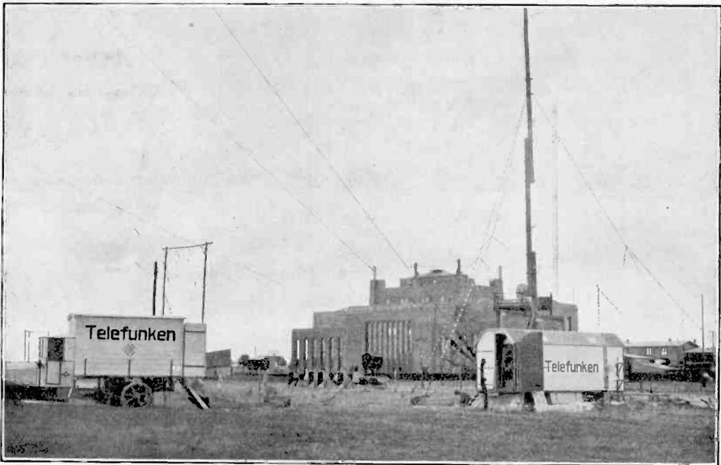
Fig. 8. *Transportable short-wave transmitter POF.*
