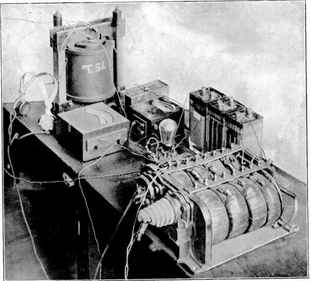
Fig. 8. Transformers and apparatus for maintaining tuning fork.
