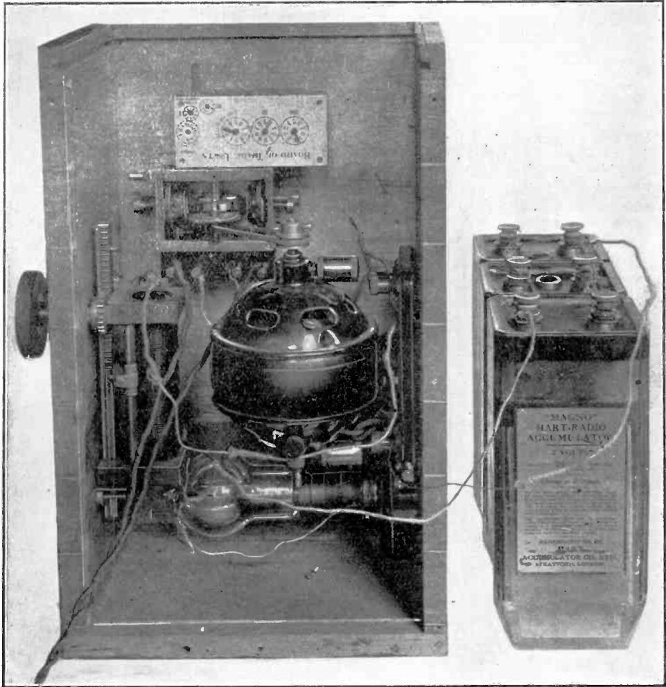
Fig. 11. *View of phonic motor, starting gear and counting train.*
