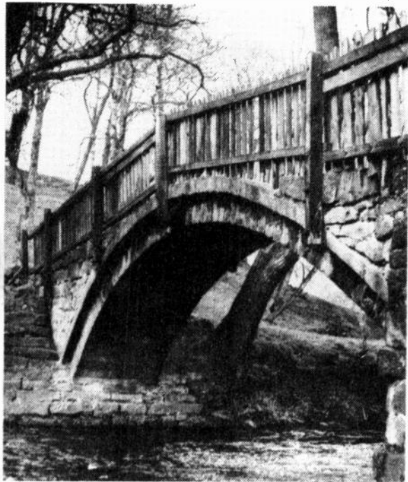
Beckfoot packhorse bridge, near Bingley, Yorkshire
