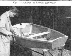
Fig. 3—Fitting rubbing strips round the gunwales
