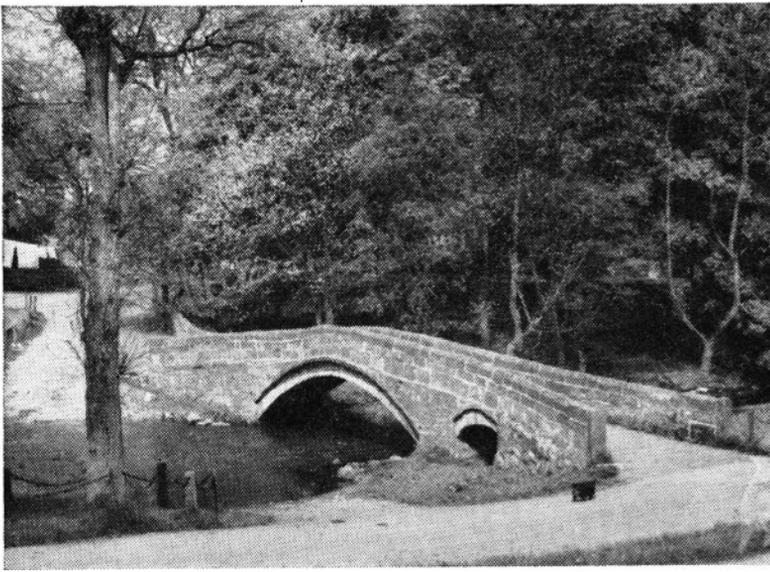
packhorse bridges were made without parapets for the simple reason that, being narrow, allowance had to be made for clearance of the wide panniers on the backs of the horses.
