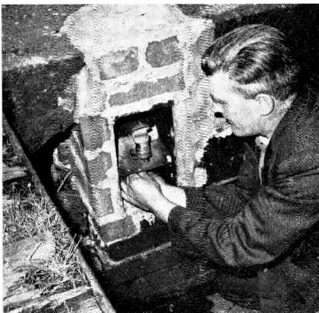
One of the ultrasonic sensing units being fitted in position
