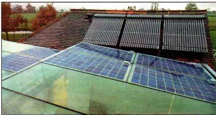
**PV Solar panels and solar water collectors**
