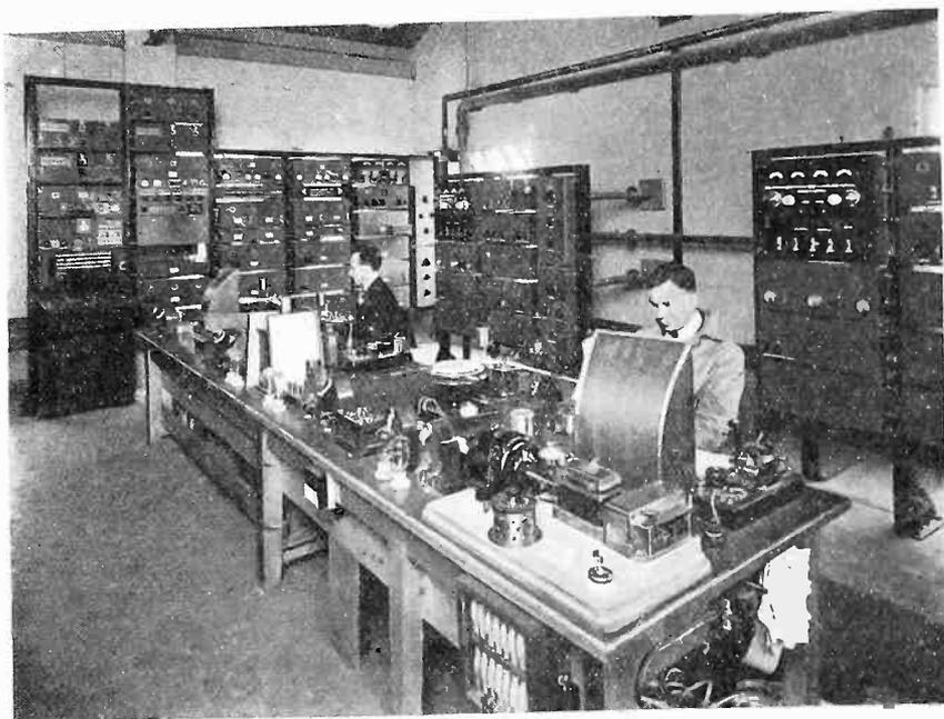
*Receiving Room at Bridgwater Beam Station showing Marconi-Mathieu Multiplex Receiver on left, and two Standard Beam Telegraph Receivers on right, with landline table.*
