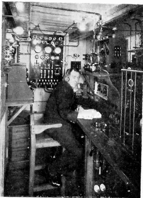
*Wireless Cabin of "Discovery," showing Marconi Direction Finder, Short Wave Transmitter and Receiver, and Quenched Spark Installation.*
