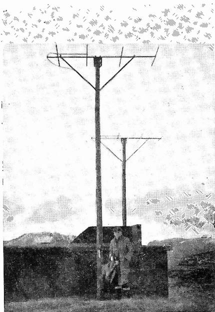
*Situated on the top of a mountain on Torshavn in the Faroe Isles a Marconi Type H.16 V.H.F. transmitter-receiver and Yagi aerial array links the telephone system of the island with those of Suderoy and Sandoy isles.*
