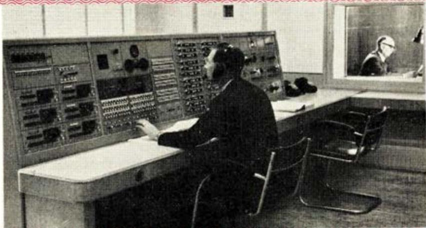
*More ambitious is the new Control Room at Bush House, London, which handles programmes for BBC's Overseas and European Services. The equipment designed by BBC engineers, provides remotely controlled switching for the connection of 150 sources to 132 outgoing routes. Programmes in the Overseas and European Services total more than 82 hours a day.*
