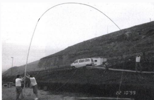
This may look disastrous, but don't panic! The Titanex 85ft-long 160m vertical is meant to bend like this. Almost miraculously, it straightens itself out and requires only one or two sets of guys.
