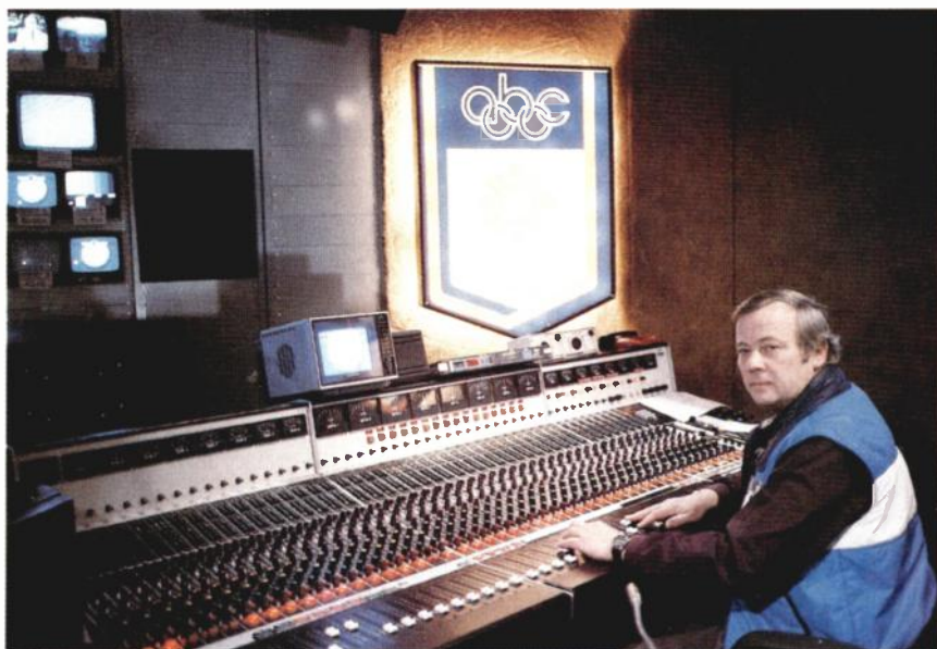
The Ward Beck audio board in Control Room A, ABC's on-air central control, is operated by Dick Roes.
