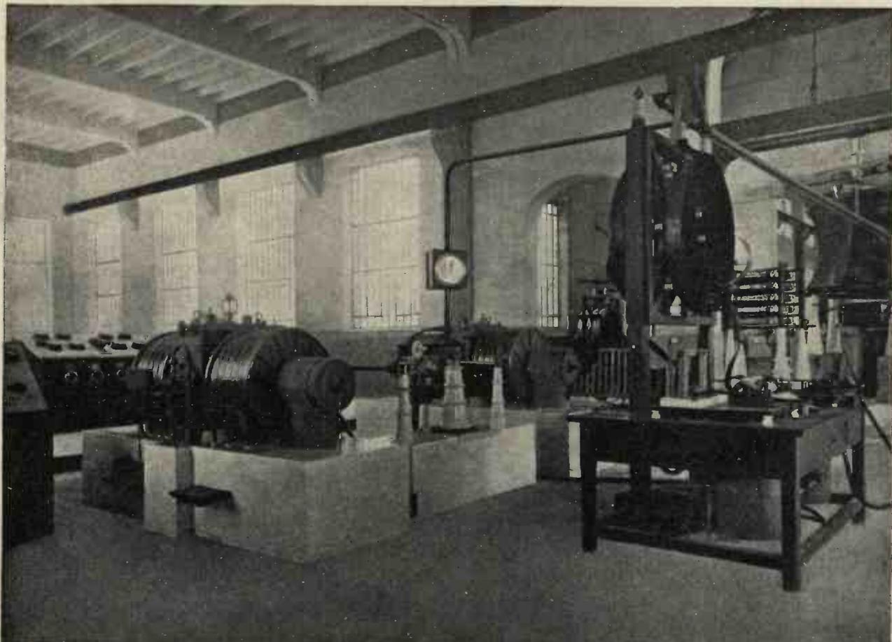
Fig. 1. Duplicate arcs installed at the Lyons station.
