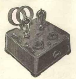
The Ethophone-Duplex is built in a one-piece matt-surfaced case moulded of an insulating compound having the appearance and properties of ebonile.
