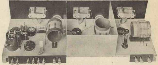
Notice how the screen is arranged and fixed by screws to the baseboard. Several of the wires passing through the baseboard can be seen in this view.
