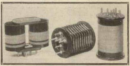
A group of typical H.F. couplings. The one on the left is an experimental "binocular" coil.
