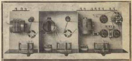
A plan view of the set, showing all the parts fixed to the upper surface of the baseboard.
