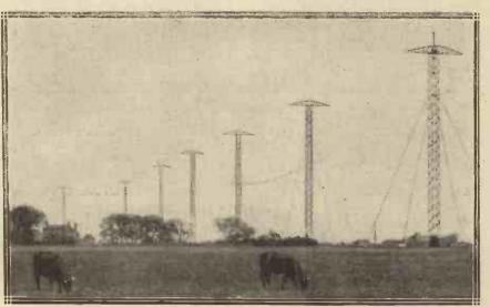
The "Beam" masts at Skegness, showing the typical cross-bar construction
