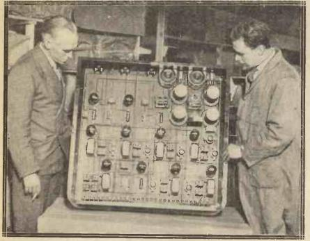
A huge wireless receiver made for St. Giles Hospital, Camberwell. It is designed to operate 550 pairs of 'phones and 42 loud speakers. The set is believed to be the largest in the country.
