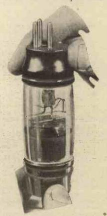
The new S.625 valve has a novel appearance. The three pins at one end are for grid and filaments, while at the other are two well-spaced pins connected to the anode and the shielding "grid." Circuits employing this valve have to be heavily screened.
