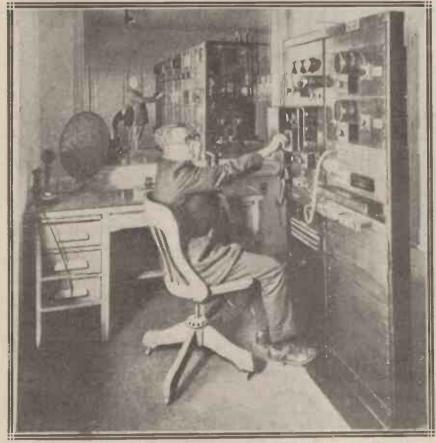
This is the control panel in the transmitting room of K F I, the Los Angeles station of the Packard Motor Co. This is the broadcaster mentioned several times by Mr. Wernerin his interesting letter. You can see the main panel in the large reflecting mirror.
