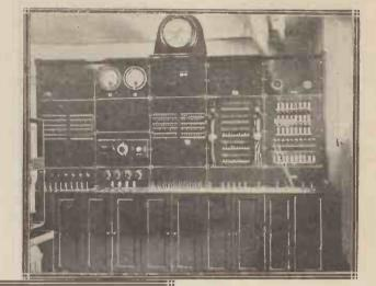
Above we have control board No. 2, which contains measuring and control apparatus for the amplifiers, the switching for outside broadcasts and lines to the relay stations. (Left) a general view of the huge new Broadcasting House.
