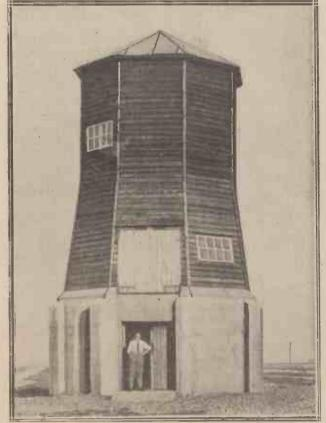
An experimental radio beacon for airmen has been erected at Orfordness, Suffolk. It sends out regular signals on "continuous" and "interrupted" waves.
