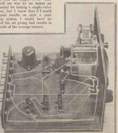
The two flexible leads in the foreground of this photograph are for the tappings on the The centre coil holder is the supplementary reaction coil. two coils.
