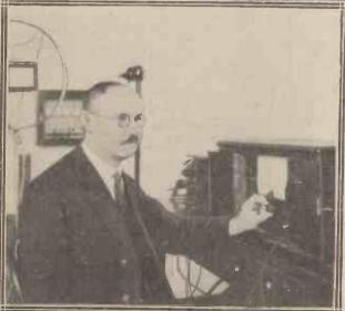
Control room 2 contains the amplifiers proper; that is, the last-stage output amplifiers. These amplifiers can be bodily replaced within a few seconds in case of breakdowns. There is a special amplifier for the loud speaker in the echo room, and one for the two loud speakers in the main studio, called the order loud speakers, as it is by means of these and a mike that the producer conveys his orders to the performers in the main studio from his special glass box in the same room.
