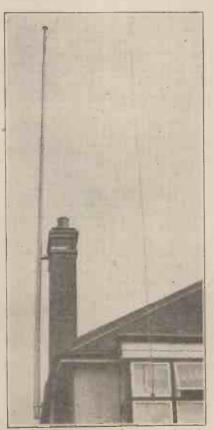
A down lead terminating in a lead-in which goes directly through the window frame. 610
