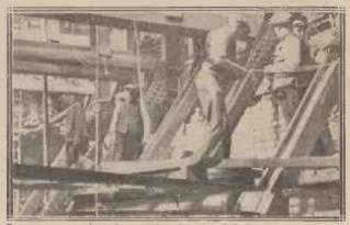
Great progress is being made with the B.B.C.'s new home in Langham Place. Here we see workmen building the steel and brick wall to hold up the road. There are to be three storeys of basement, the building itself being twelve storeys high.
