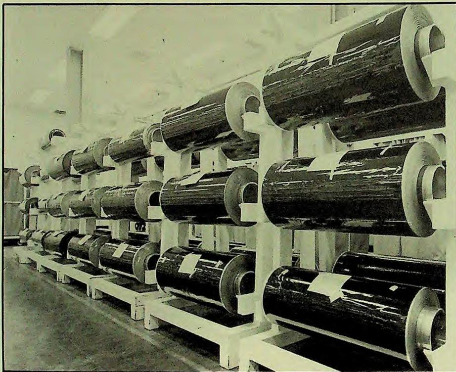
JUMBO ROLLS of tape await slitting at 3M's Gorseinon plant. Mass production, with the heavy investment needed to meet the new mass market for blank video tape, has boosted quality, say factory management.
