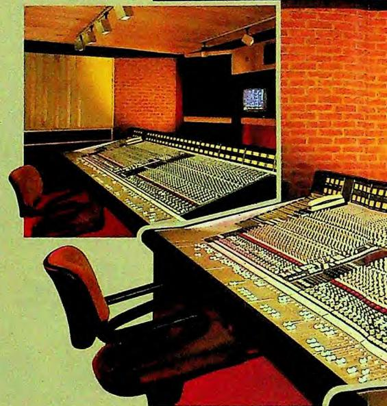
Battery Four, operational since November 1984, houses a 48-channel SL4000 E Series console, computer-assisted and with Total Recall. During remix, the small faders may serve as additional line inputs, allowing Battery Four to handle as many as 96 simultaneous sources!
