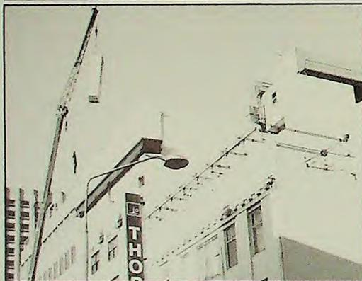
SYDNEY: Installation of a new Solid State Logic console at EMI's Studios 301 meant that a hole had to be punched in the eighth floor roof in order to lower the one tonne console into position.
