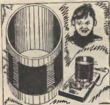
Coils for Crystal Sets. Consist of 70 turns, 24-gauge D.C.C. Wire on 3in. diam. bakelite former. Tapped every tenth turn.
