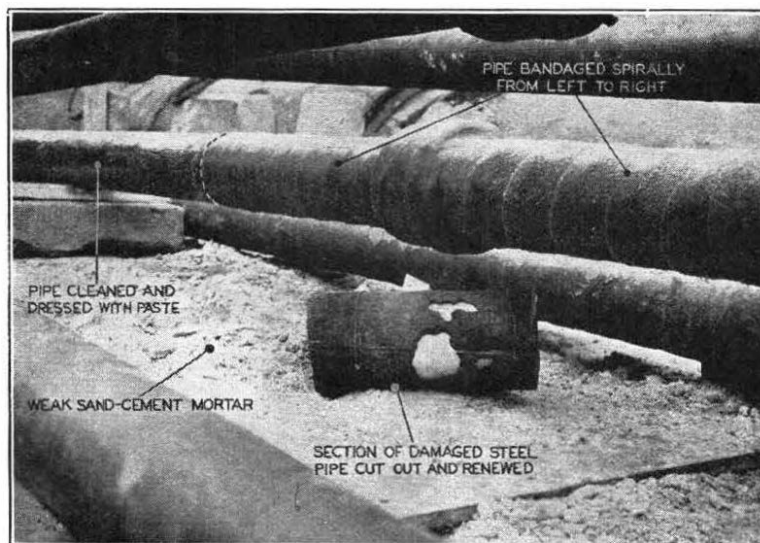
FIG. 4.—P.O. PIPE UNDER TREATMENT.
