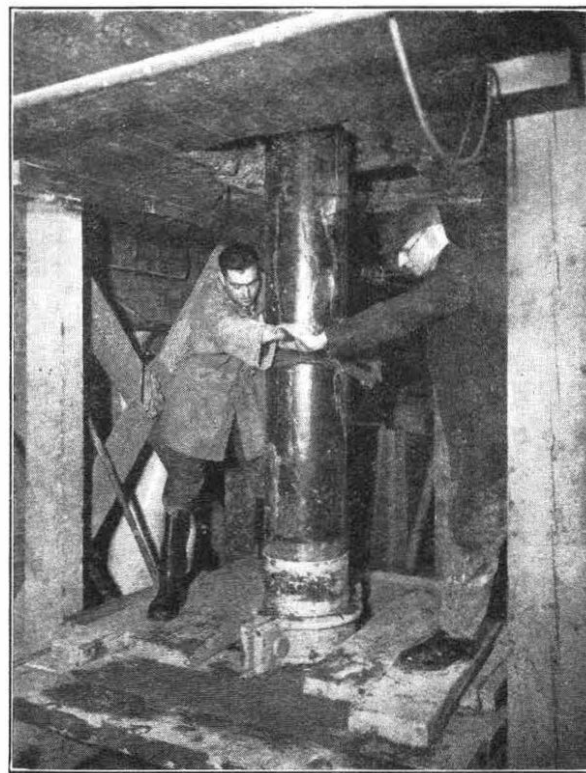
FIG. 2.—SCREWING IN A SECTION OF BORE TUBE.
