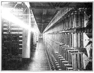
FIG. 7.—ILLUMINATION OF LOWER PART OF M.D.F. WITH MEZZANINE PLATFORM, USING FLUORESCENT LIGHTING WITH CONTINUOUS REFLECTOR.
