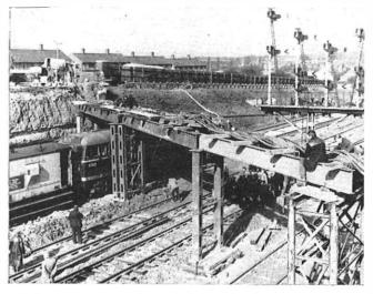
SUPPORT FOR POST OFFICE CABLES AFTER BRIDGE COLLAPSE
