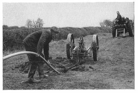
FIG. 7-CONTROLLING ANGLE OF DUCT ENTERING PIT
