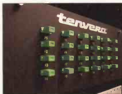
Head-end distribution board with posts to hang fibre reels
